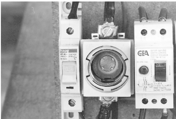
Fig. 4.21 Earth leakage circuit breaker
