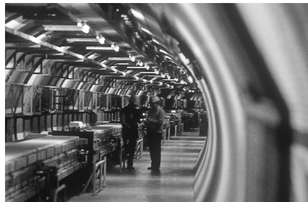
Fig. 1.5(b) Inside the LEP tunnel (Photo CERN)
